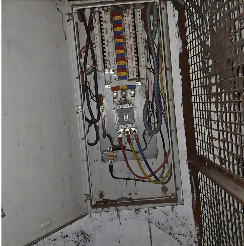
Image 3: Exposed electrical panels right in the middle of leather storage
